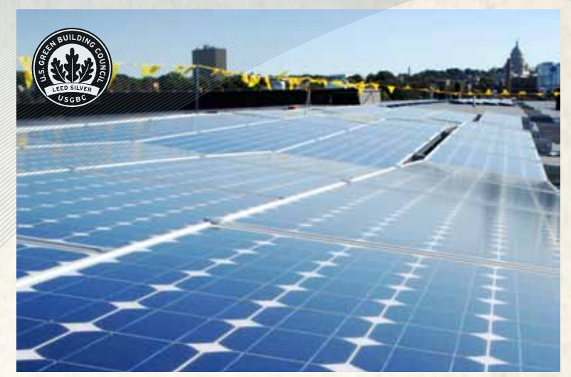
9. Providence, RI LEED® Silver Certified, featuring a 142 kilowatt solar panel array
